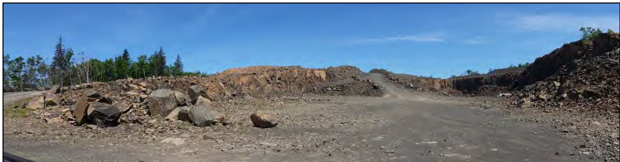
Figure 2. North view of Seabrook Quarry, June 2015.
