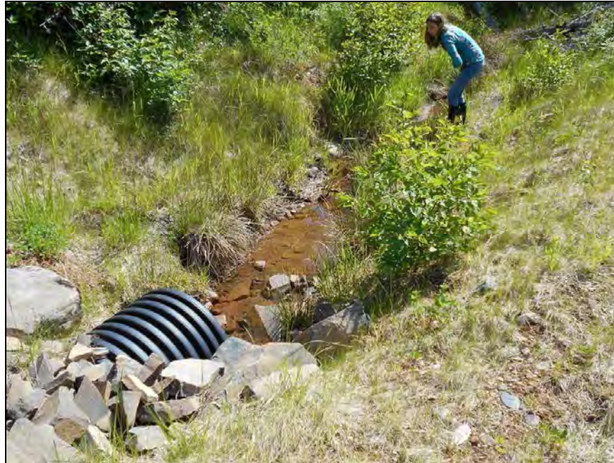
Figure 23. Downstream view of one of the ditches draining the part of the steep area of the access road, June 18, 2015. Flow is to the southeast.
